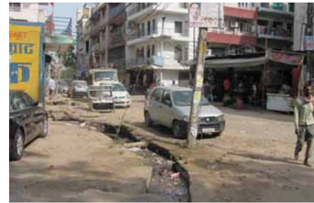
Open drains filled with sewage
