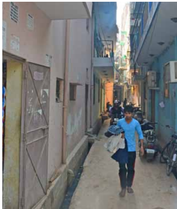
Unconnected drains filled with stagnant sewerage
