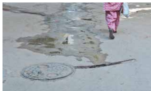
Connections in sewer lines transferring surface water
