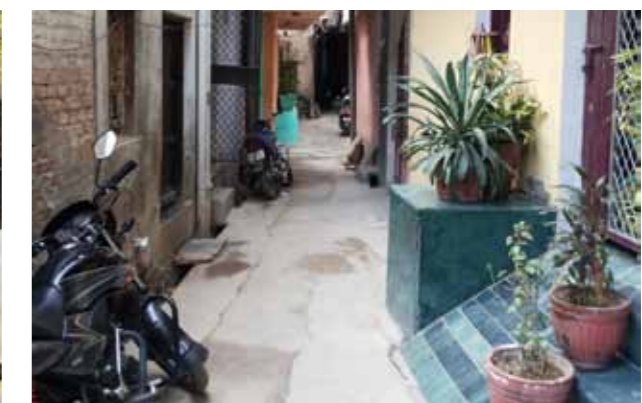
Backward sewerage flow and rain waterlogging
